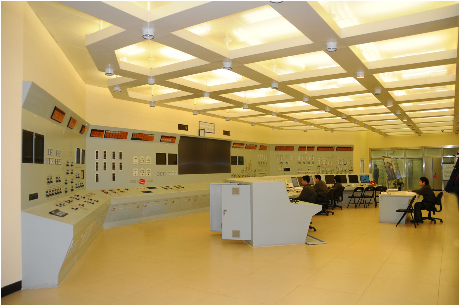
Main control room (2009.01)
